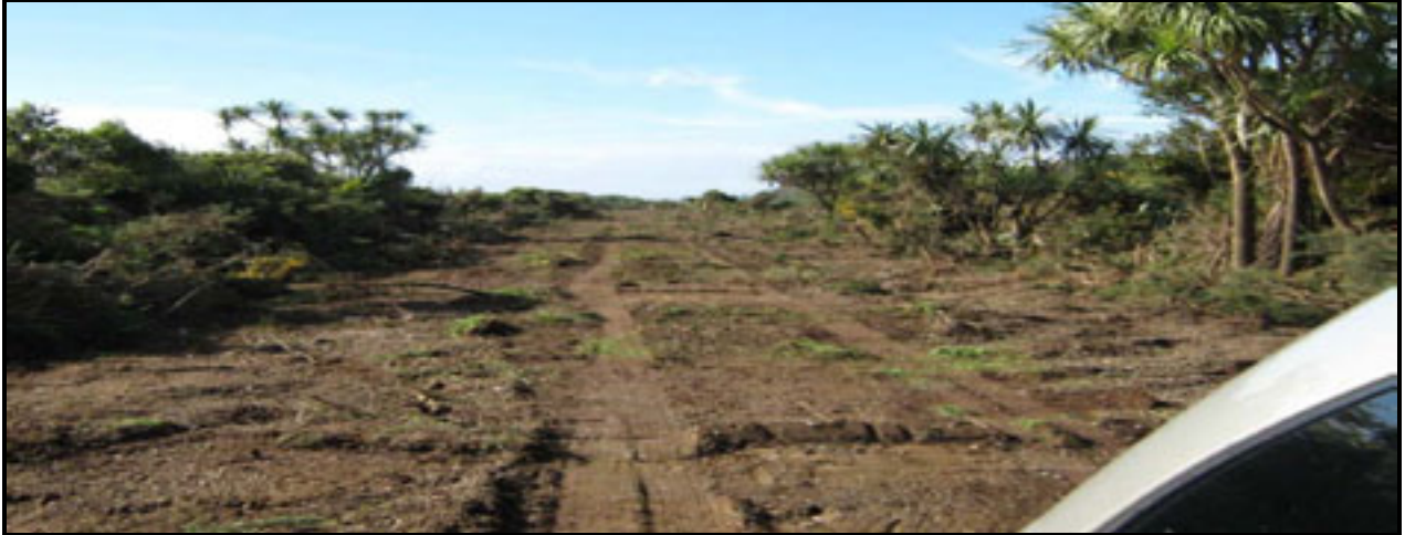
Figure 7: A portion of the clearing carried out.
