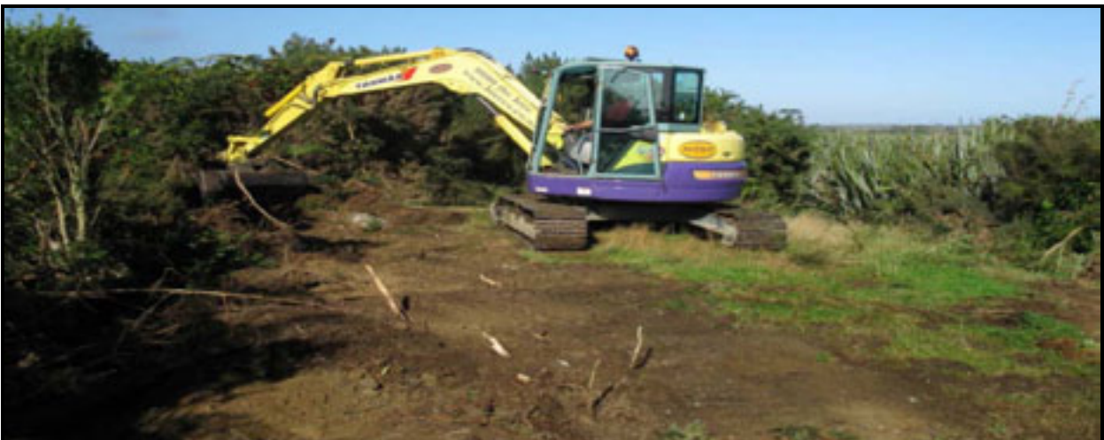
Figure 8: Machine working on mineralised strand line
